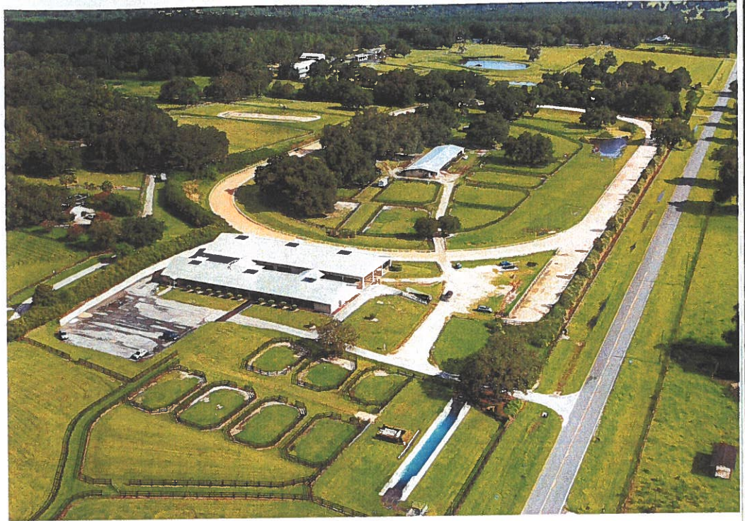
The Equine Performance Innovative Center near Ocala, Fla., has stall capacity for 42 horses, including two 20-stall barns and a special area in a climate-controlled therapy building with air-conditioned and heated stalls.
